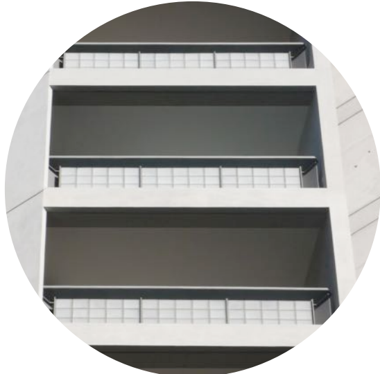
steel frame balustrade, glass block infill
